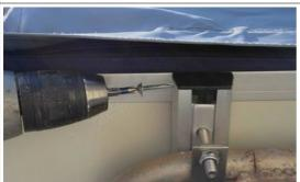
Add the end caps and secure them in place with self drilling screws.
